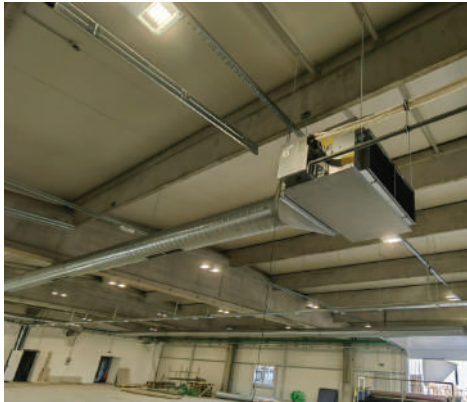
Roundliner BR Prijedor, BiH VMV S System capacity: 2 x 28.0 kW
