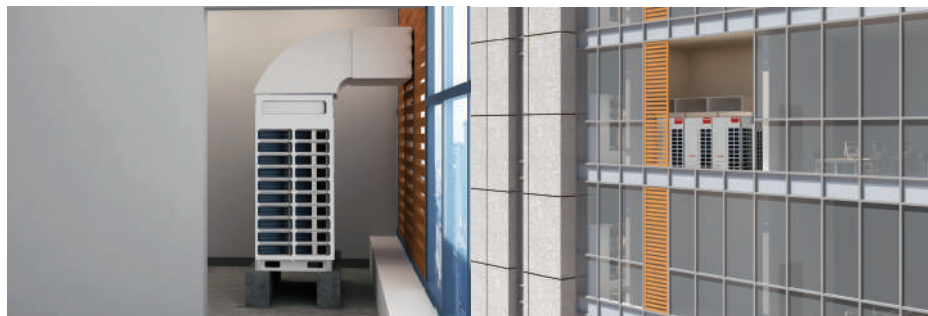
Installation of duct
